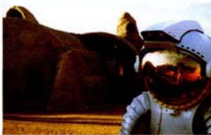
Cal-Earth Institute's "Earth One" prototype structure was constructed and tested using unstabilized superadobe/superblock walls. Cal-Earth prototypes are also used as grounds for space suit maneuvering and documentary research.
