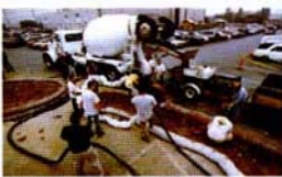
Superadobe/superblock coils under construction, demonstrating pumping method.
